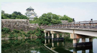
K Gokurakubashi Bridge
