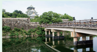
K Gokurakubashi Bridge
