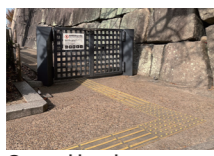
Ground level elevator entrance
