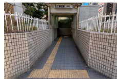
Tanimachi Line Temmabashi Station elevator
