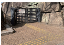
Ground level elevator entrance
